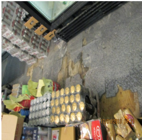
10) Flooded and very poorly maintained flooring areas.
